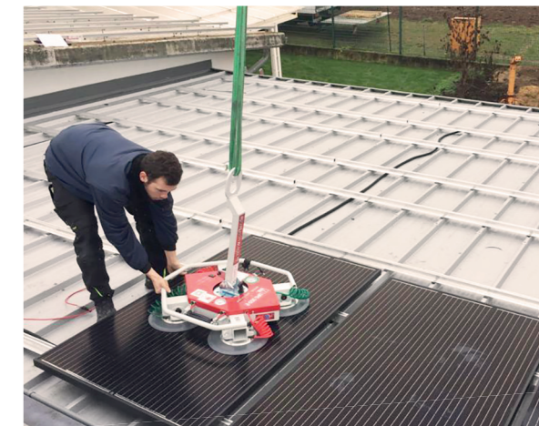
The UPG350 can suction elements such as solar panels, veneered wood, metal and plastic panels and much more
